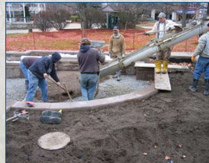
Workers from Country Farms construct Scottdale Library Rain Garden
